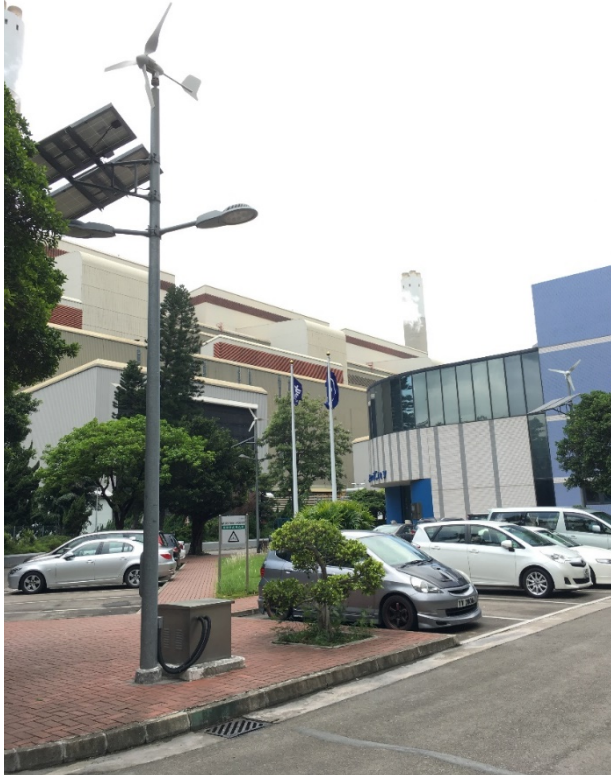
Figure 2. Series of wind turbine poles with solar panels at a power generation station in Hong Kong.
