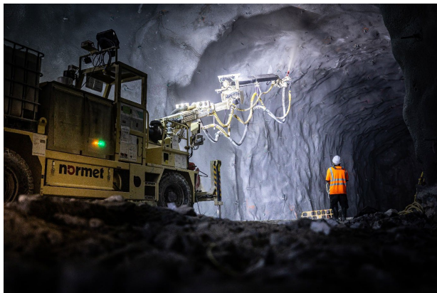
Figure 2. Shotcreting inside Sha Tin cavern.
