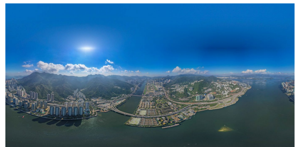
Figure 9. General view of the project site.
