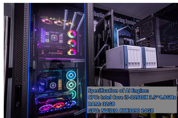
Figure 3. AI engine for overbreak prediction in the AI room at Sha Tin cavern's site office.
