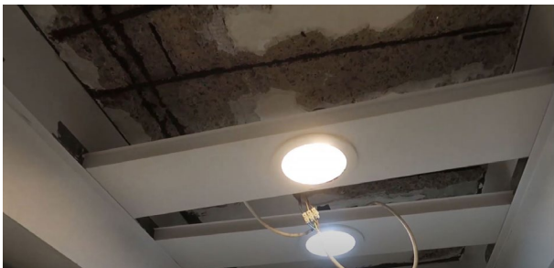
Figure 6. Examples of carbonation-induced damage. (a) Wide cracking in a bedroom; age of building = 28 years; (b) local spalling in a bedroom; age of building = 28 years; and (c) widespread spalling in a washroom; age of building = 38 years.
