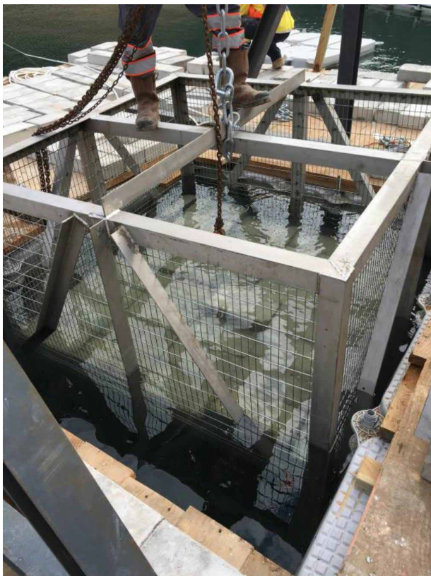
Figure 3. Assembly of a gravity anchor at Shek Pik Reservoir comprising a steel cage packed with small concrete blocks.
