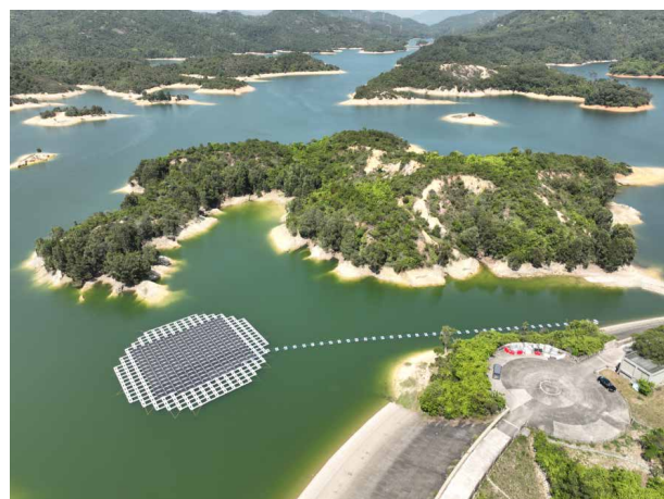
Figure A3. FPV system at Tai Lam Chung Reservoir.
