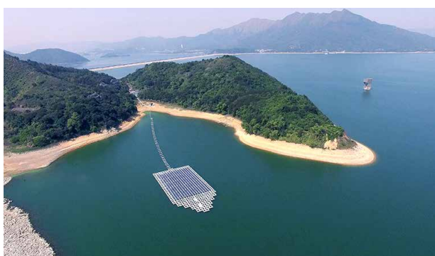
Figure A2. FPV system at Plover Cove Reservoir.
