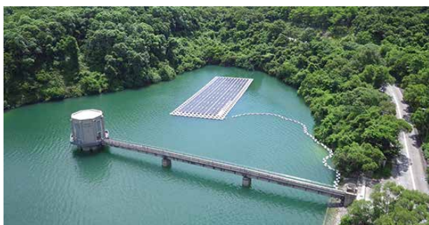
Figure A1. FPV system at Shek Pik Reservoir.
