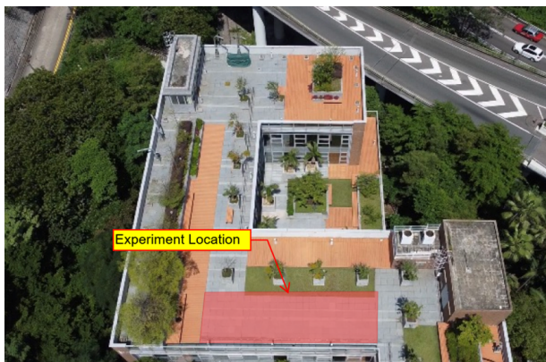
Figure 5. (a) 3D satellite view of the project building; and (b) 3D satellite view of experiment location.
