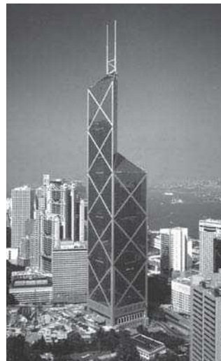
Figure 13 – The Bank of China Tower: Overview
