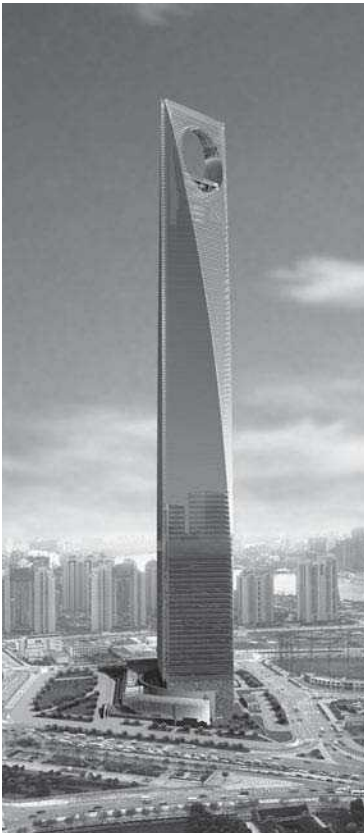
Figure 20 – Shanghai World Financial Centre: Overview
