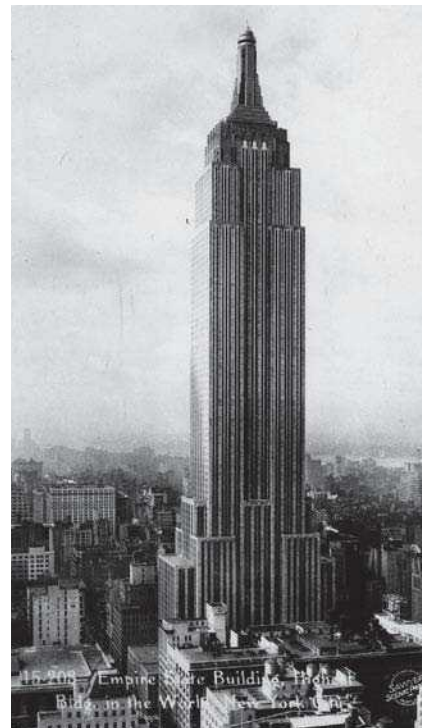
Figure 1 – The Empire State Building
