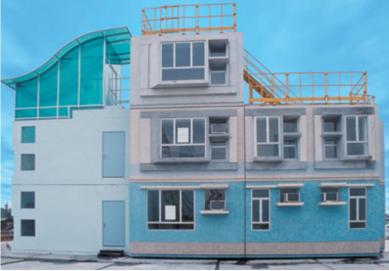
Fig 2. Stacked modules, complete with windows, tiles and air-conditioner reeves
